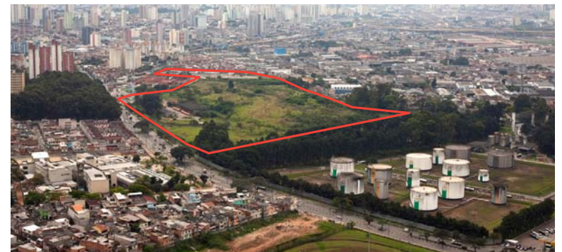
Aerial view of the site from the south-west
