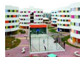
2. Gleba H, 162 units, completed 2011
