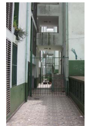
Gates installed by Gleba A residents to create smaller unit clusters
