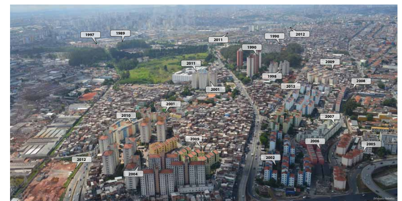
Aerial view of Heliópolis from the north-west illustrating COHAB interventions
